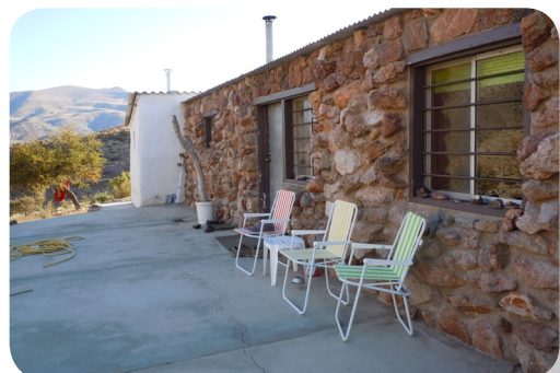
Volunteer Housing - The Adobe
